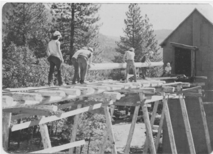
Trestle Work, April, 1976.
