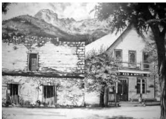
The stone building, thought to be the Columbo Saloon.
