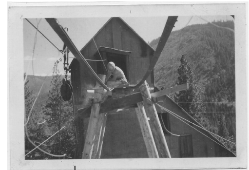
Trestle Work, April, 1976.
