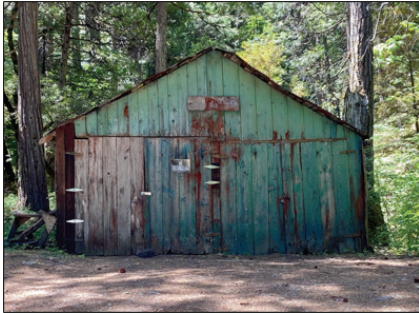
Outbuilding on Crow City Road (Photo by C. Jimenez).
