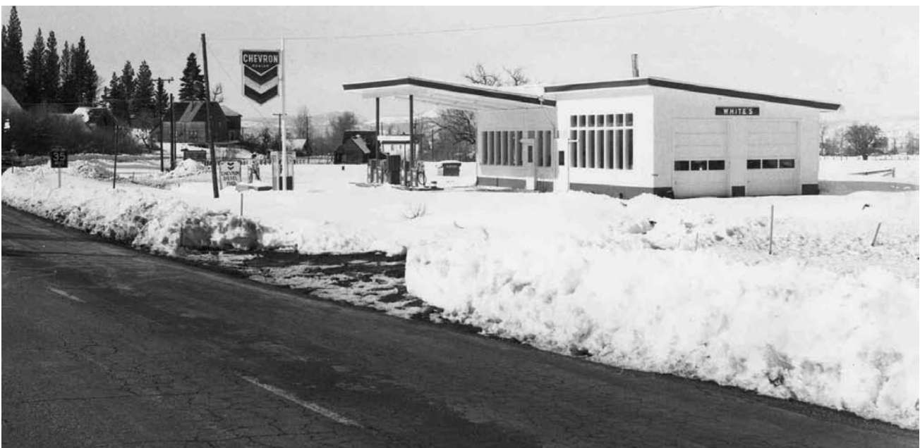
Ed's Sierraville Service Station
