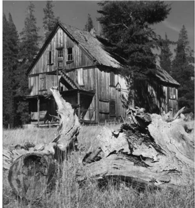
The old apartment house.
